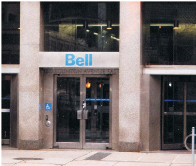
Bell Canada in Toronto one of the City Multi installation sites in Canada.
