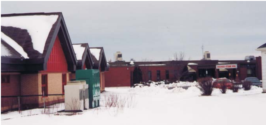
Ridgewood veteran wing is air-conditioned with four City Multi (VRF) systems.
