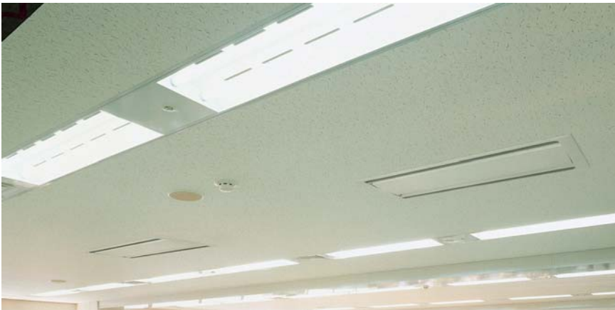
Two way diffusion ceiling cassette units where used at Ridgewood Veterans Wing.
